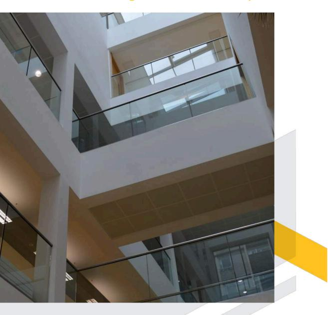
Atriums, bridges and walkways can give a building a sense of space and allow buildings to be flooded with light. It's imperative that along with this style, comes a heavy-duty guarding able to deal with potential overcrowding and heavy traffic.
