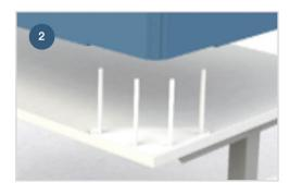
The panel is drilled to a line with the spigots.
