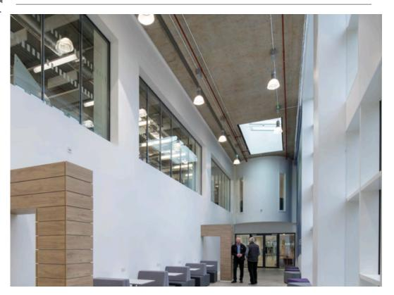
Polar Double Glazed FR is ideal for when stringent fire and acoustic requirements apply, achieving up to 30/0 fire rating. Alongside its discreet framework, this system combines contemporary aesthetics, performance and durability.
